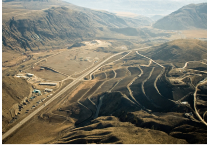
Aerial view of the Cache Creek regional landfill.
