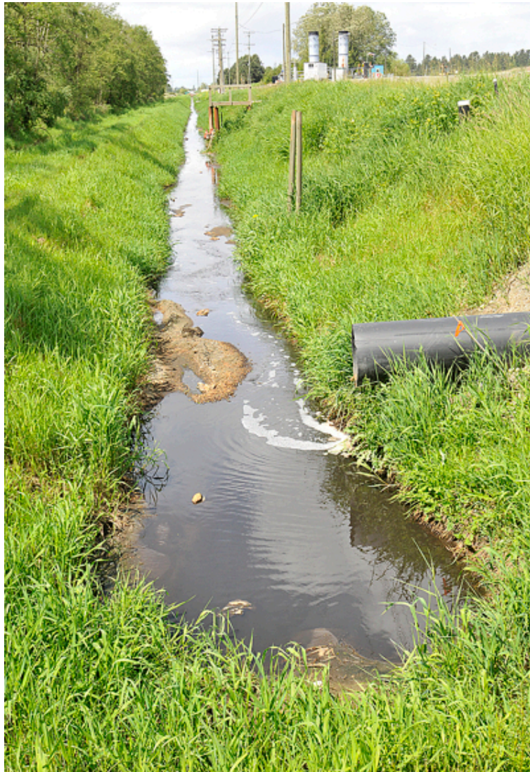
Landfill gas is collected from the Vancouver Landfill. Some is flared off at on-site burners (top) but most is piped to nearby greenhouses to create electricity and heat. Dikes (above) surround the landfill and trap leachate, which is then sent to a sewage treatment plant. Photos: Evan Seal / The Leader
