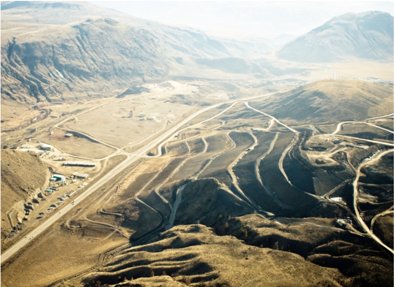
Aerial view of the Cache Creek Regional Landfill. About a third of Metro Vancouver's garbage is trucked 350 kilometres east to the site, which accepts up to 500,000 tonnes per year and is slated for expansion. Photo: Arnaldo Rodriguez
